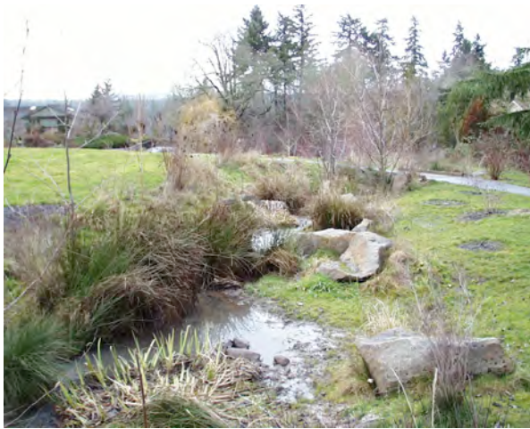
Photo 16. A daylighted storm drain (1994) Freepons Park, Lake Oswego Once a storm drain Now a natural stable stream Freepons Creek drains to Oswego Creek
