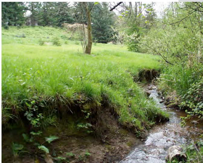
Photo 3. Severe stream bank erosion Springbrook Creek
