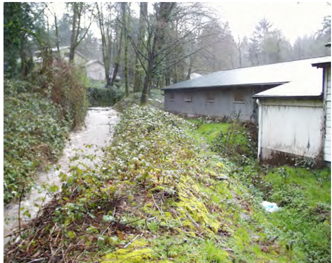
Photo 11. Potential flooding hazard, degraded aesthetics, & loss of habitat Springbrook Creek
