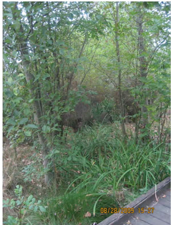
Photo 16. A daylighted storm drain (2009) Freepons Park, Lake Oswego 15 years later
