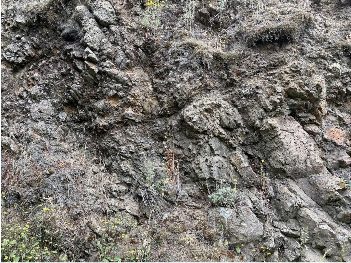
Figure(2). Here are two photos demonstrating project site at a higher elevation.
